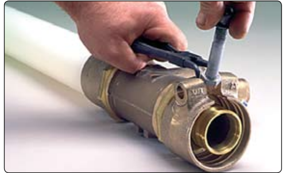
Figure 6: Insert Bolt Head
