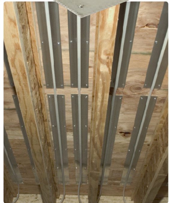
Wirsbo hePEX tubing easily and securely snaps into the Joist Trak channel for faster installations without extra fasteners.
