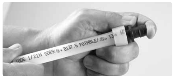
Figure 3-10: Insert Fitting into Tubing
