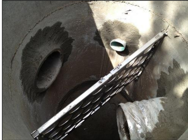
The SAFL Baffle is a cost-effective method to help cities treat urban runoff that goes into storm sewers and eventually ends up in lakes, rivers and oceans.
