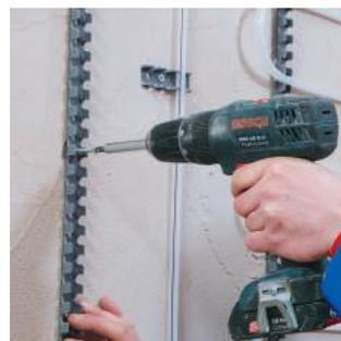
*The Uponor Fix wet plaster systems can be installed simply and rapidly with the practical system accessories.*
