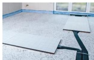
*Uponor Comfort Air is installed together with the Pluggit Pluggflex ventilation ducts. The corresponding adapters enable professional integration into the ventilation system.*
