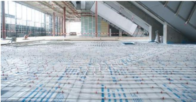
The Uponor Classic wet construction system contains all the components that are required for practice-oriented laying on the building site. Corrosion-protected bearer elements and Uponor Classic pipe holder for the basis for precise positioning of the Uponor Comfort Pipe PLUS heating pipe. The 0.2 mm thick, robust Uponor Multi Foil offers protection against moisture from the screed as a insulating layer cover in accordance with DIN 18560.
