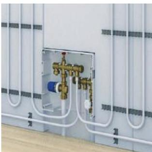
*The compact Uponor Minitec connection box is integrated into the wall structure and offers direct connection possibilities for up to three heating circuits.*
