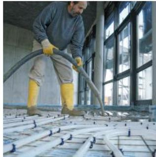
**Uponor Classic wet construction system is the ideal underfloor heating and cooling system for variable flooring structures in new residential building construction and in the commercial field. Three different mat grids make optimal adjustment of the heating pipe spacing to the respective heat requirements possible. In combination with high-load insulation materials the Uponor Classic wet construction system can also be used in areas subject to high service loads.**
