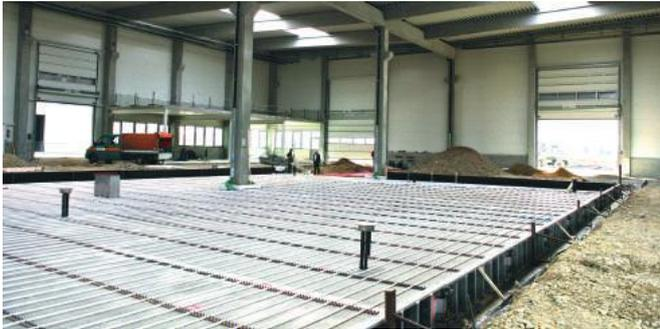
Industrial floor heating are integrated into the structural element and are practically maintenance-free. In addition, no scaffolding or elevating platforms are needed, in contrast to ceiling systems. Even manifolds are not required if the terminating piping is laid within the industrial floor and the connection to the heating circuits is carried out in accordance with the Tichelmann (reverse return) principle. Uponor disposes of the required special know-how.
