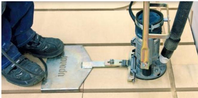
The Uponor Calma components ensure a smooth and easy installation process that is fully compliant with all relevant construction norms and regulations. The pipes are positioned and fixed in place in the heat emission plates. These features not only ensure that heat output is transferred exactly as calculated, they also enable precision temperature control and lead to substantial savings on energy and operational costs.
