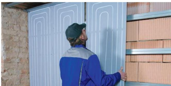
**The Uponor Renovis radiant heating/cooling system consists of a gypsum plasterboard in which the Uponor PE-Xa pipes have already been integrated in the factory. It allows the temperature control of rooms via walls and ceilings in dry mortarless construction. An extensive Uponor range of products is available for professional interconnection of the panels in accordance with the Tichelmann principle.**
