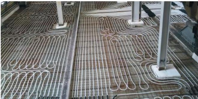
With Uponor Magna heat is available where it is needed, namely in an area up to approximately 2 m above the heated flooring. This is an advantage in particular at high halls as heat does not accumulate in the higher areas like it is the case with air systems. Therefore, the heat loss via the ceiling can be minimised.
