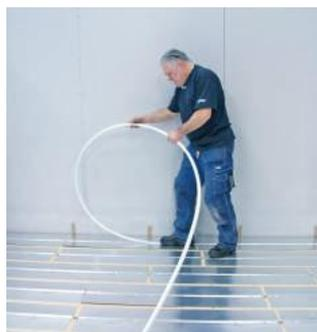
**Uponor Calma is an underfloor heating system specially developed to give extra sound reduction. This system is installed directly on an existing floor, and is therefore suitable for renovation purposes where there is no limitation in maximal floor thickness.**
