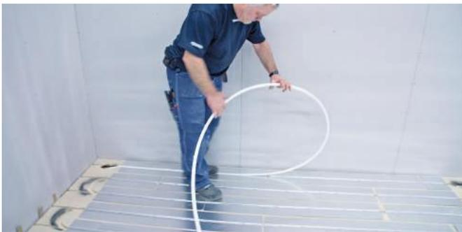
**Uponor Tignum is used for quick installation on joist directly in a timber floor approx. 600 mm. It is flexible to use since it is suitable for many "on joist" floor constructions.**
