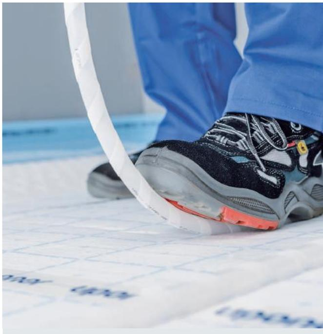
Uponor Klett can be laid rapidly and simply. The pipe is laid either manually or rolled of from by the practical mobile Uponor pipe winder and placed on the laid systems boards. The printed-on laying grid serves as an orientation aid for even pipe spacings (10 x 10 cm). Special laying or fastening tools are not required.
