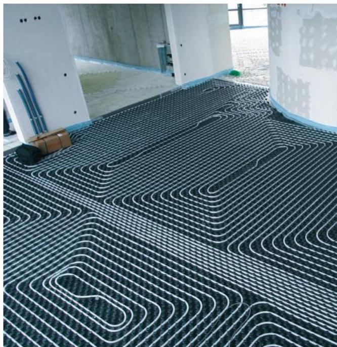
The Uponor Tecto wet construction system can be laid by a single person. The size of the nub panels of 1,450 x 850 mm guarantee high laying performance.
