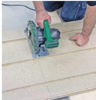
Just a few components for a fast installation: panel, turning plate, multi heat emission plate extra and heating pipe. Use the Uponor milling machine to make grooves or use specially made turning plates. The panels are easily cut with a circular saw. The plates are easily divided by bending them only. The pipes are positioned and fixed in place in the heat emission plates.
