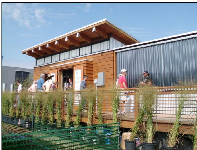
The winner of the 2011 Solar Decathlon, the University of Maryland's WaterShed House, features an Uponor crosslinked polyethylene (PEX) plumbing system.
