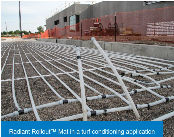
Radiant Rollout™ Mat in a turf conditioning application
