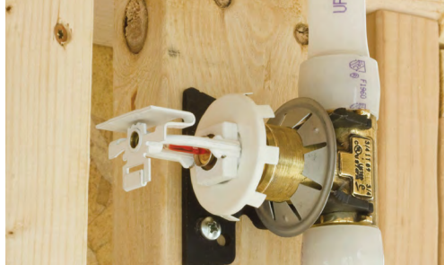
Figure 1-7: ProPEX tee with horizontal sidewall sprinkler
