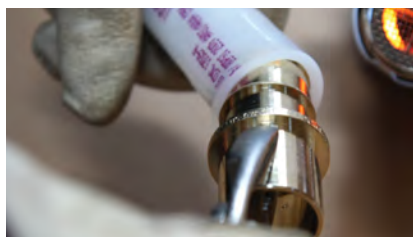
Figure 7-36: Work piping back and forth
