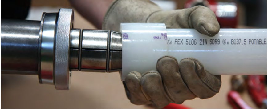
Figure 7-22: Slide head into piping
