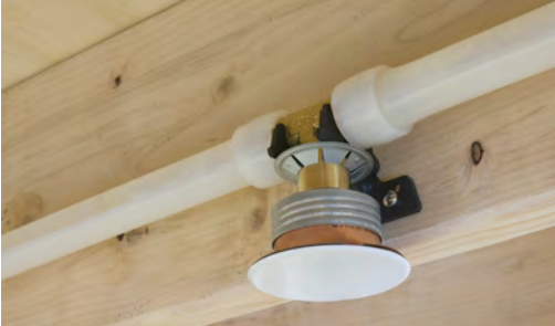
Figure 1-6: ProPEX tee with concealed sprinkler head
