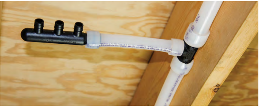
Figure 8-1: Feed plumbing fixtures via EP multiport tees
