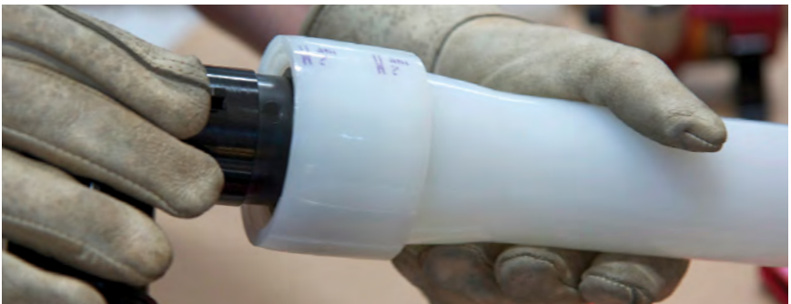
Figure 7-26: Insert fitting
