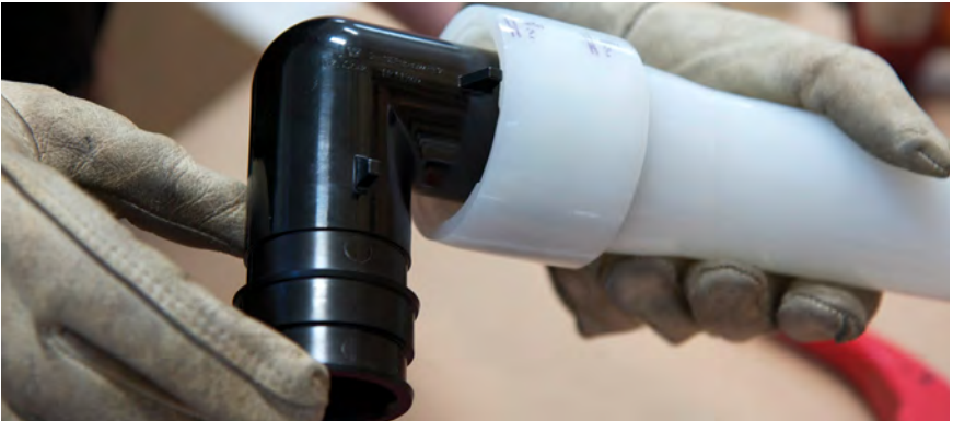
Figure 7-27: Ensure piping and ring seat against shoulder of fitting
