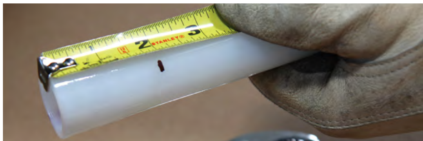
Figure 7-38: Measure from end of pipe
