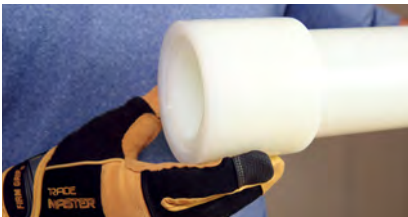
Figure 7-16: Ensure ring reaches stop edge
